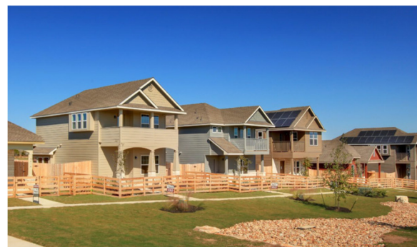
The developer of Whisper Valley in Austin, Texas mandated that all structures in the entire
